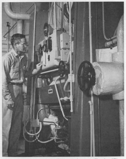
ABSORPTION REFRIGERATION unit for controlling humidity, temperature in IBM 705 area is checked by James Skidmore (4511).
